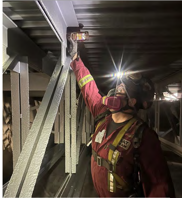
Tacten Coatings Inspector Inside Coal Silo Four
