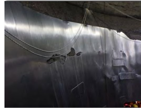
Silo plates prior to replacement
