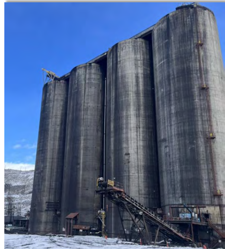
Coal Silo Number 4
