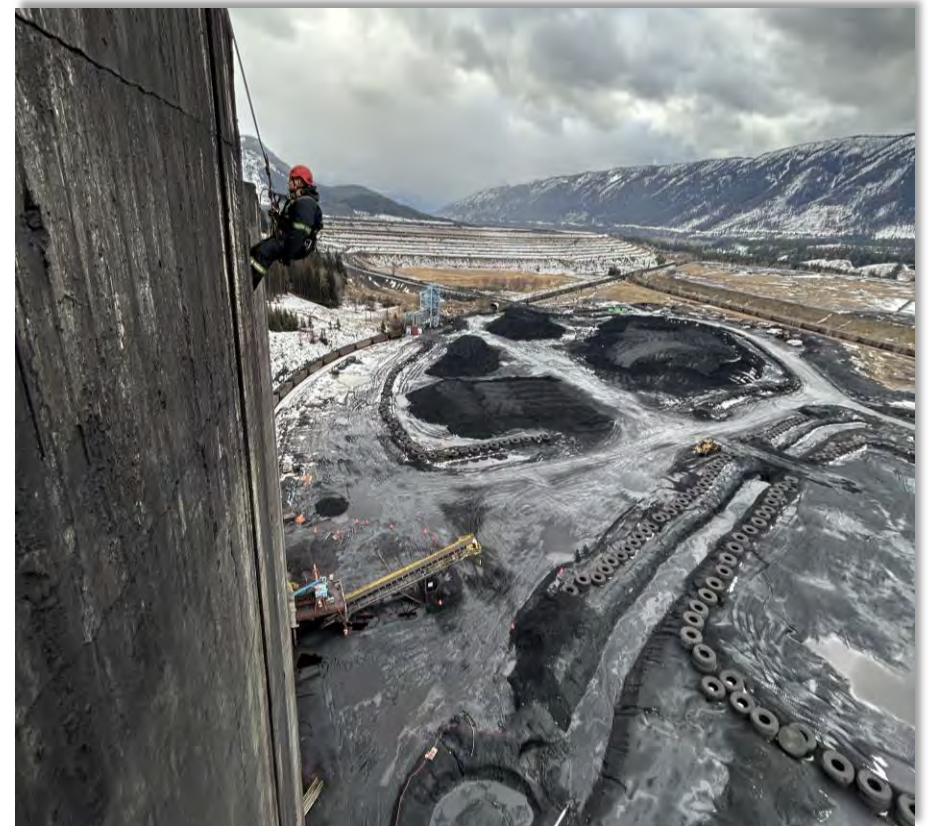
Rope Access Technician on the Side of Coal Silo
