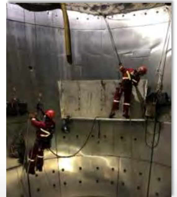
Tacten crews completing plate replacement
