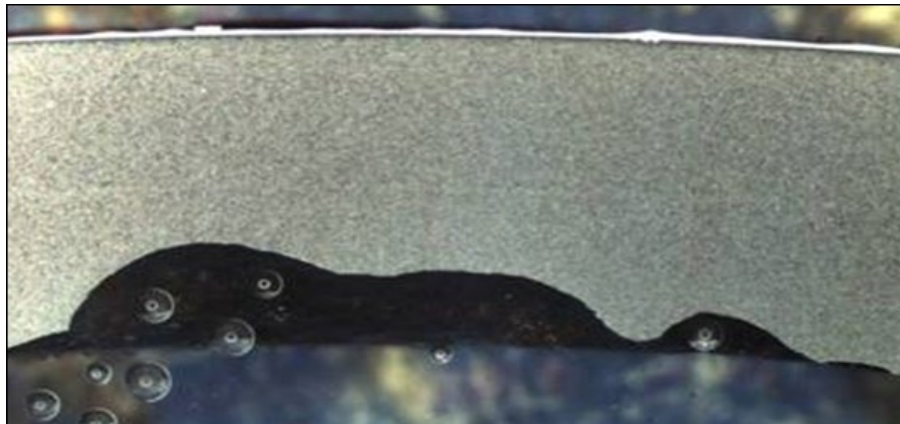
Figure 5. Cross-section of galvanized pipe shows the severe nature of the internal pitting.
