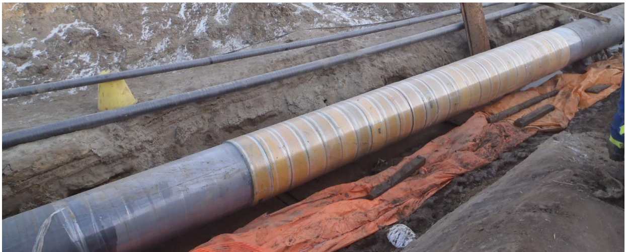
Figure 2. The 34" natural gas pipeline after the repair.
