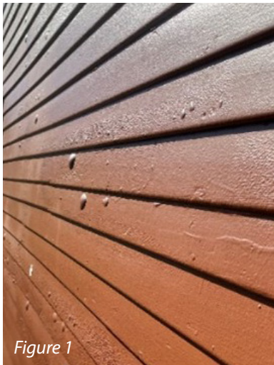
Figure 1: The paint blisters as they appeared on the siding. Figure 2: An opened blister reveals bubbles underneath the coating. Figure 3: A macrograph (~64x magnification) showing bubbles present throughout the primer layer.
