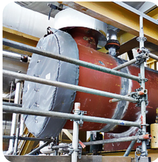
Sulfur condenser located in a sweet and sour gas processing facility
