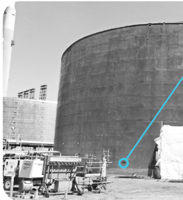
Insulated tank with insulation perforations acting as paths for moisture ingress
