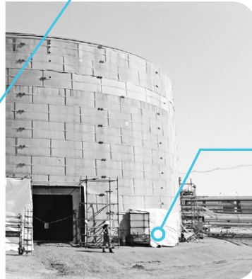
Tank with insulation removed and exposed CUI damage
