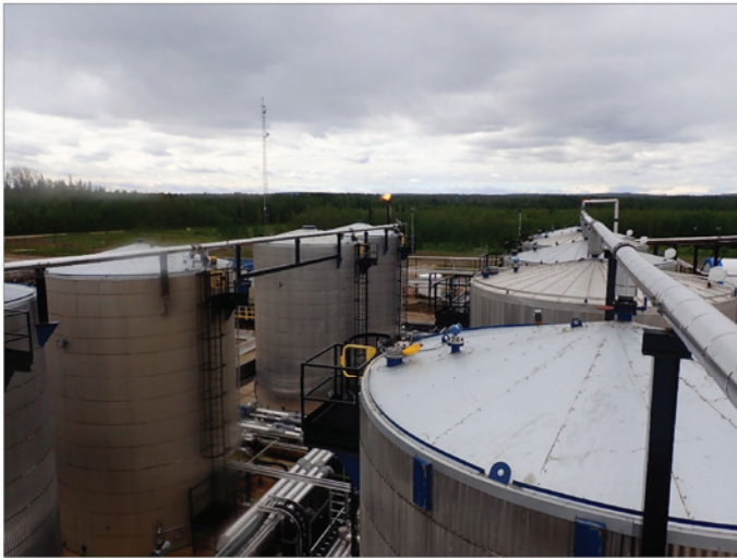
Figure 1. Overview of the tank farm.
